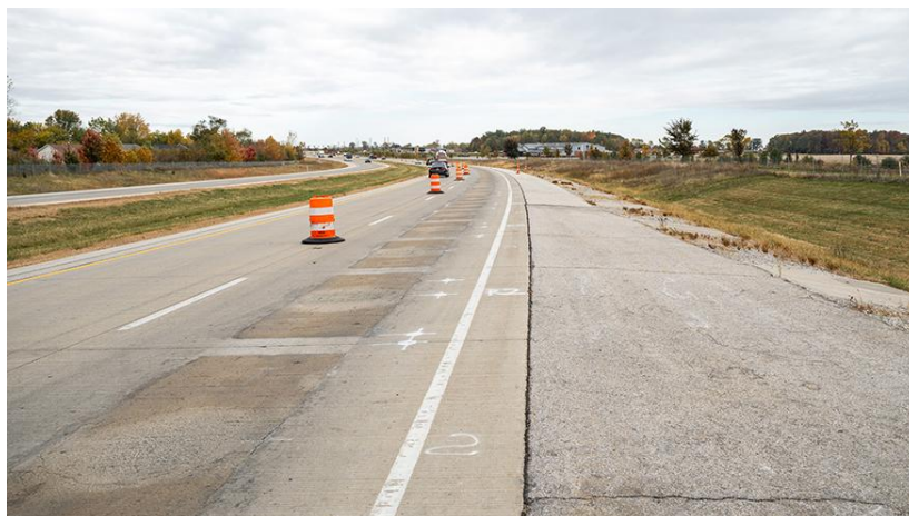
Rectangular receiver pads are visible in the lane that an electric truck equipped with receiver coils would use to charge as it drives. (Purdue University photo/Kelsey Lefever)
