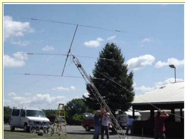
Tower Raising at New Germany Grove
